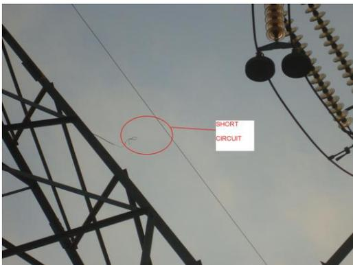
Fig. 4. Induced Short-Circuit on Transmission Line
